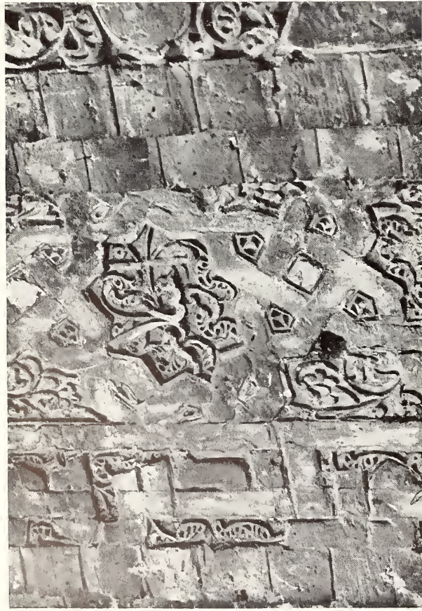
PHOTO, M. B. SMITH, NEG. L-320 FIG. 28—MIHRĀB, CAVETTO OF FRAME, DETAIL OF BRICK-GAČ REVETMENT
